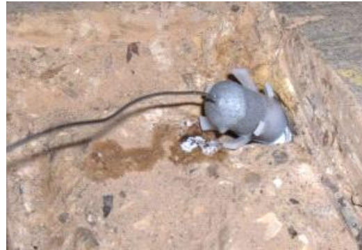
Figure 1 Installation of a galvanic anode at an area of concrete repair.
