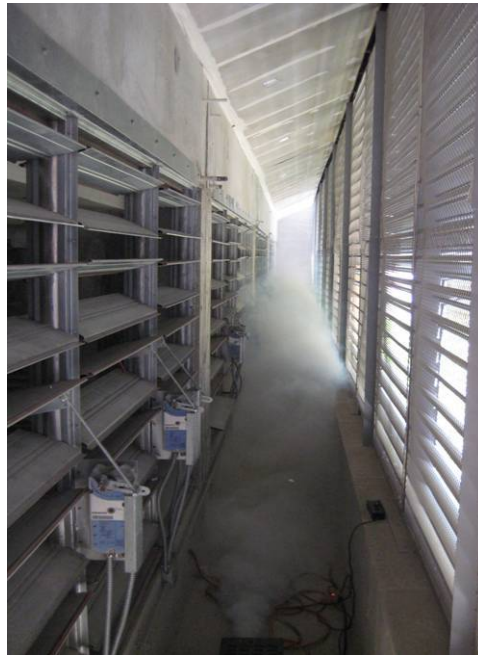
Fig 8: Louvered air inlets on SE side of the library
