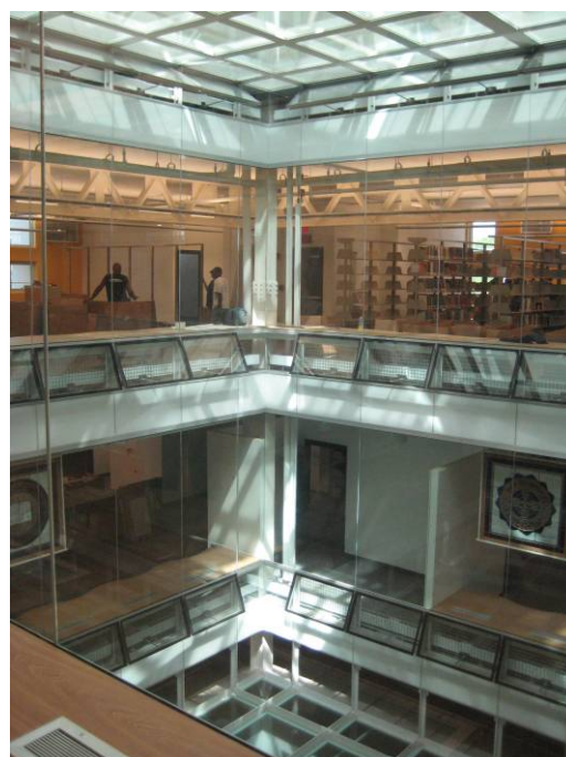
Fig 4: Lightwell, glazed floor, horizontal glass lens, air inlet slot from plenum and air outlets to each level
