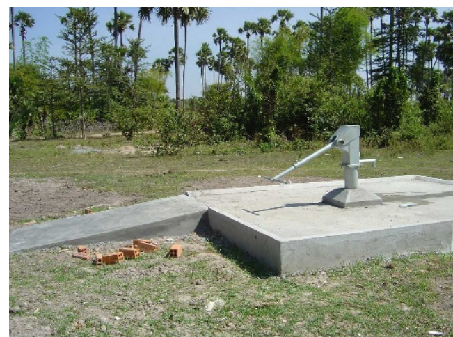
Figure 2. Handpump platform with ramp in Cambodia
