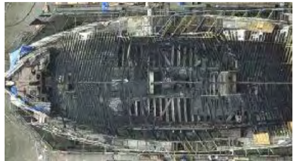
Cutty Sark Fire, 2007 The remains after the fire
