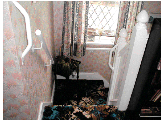
Figure 4.4 Grab rails on stairs (household 133)
