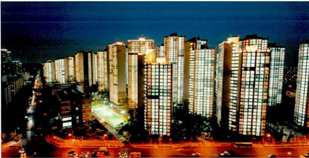
Figure 6-4: The Park-Rio Apartments in Song-Pa Gu Area (on 21 st July, 2008)
