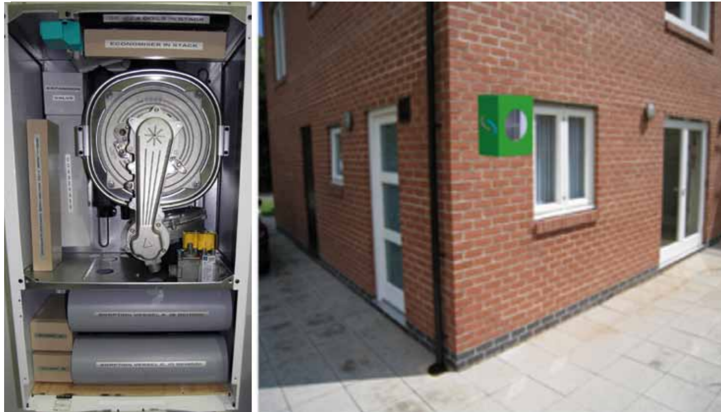
Figure 1: Illustration of CALEBRE gas-fired heat pump (developed at Warwick University)
