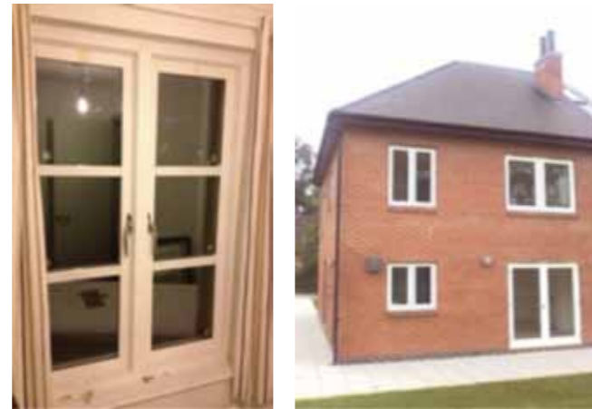
Figure 5: Vacuum glazed window in E.ON test house
