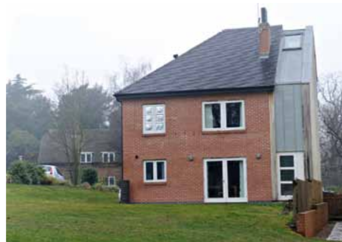
Figure 1: The E.ON Retrofit Test House which is being used to trial CALEBRE technologies
