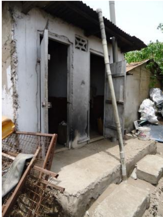
Figure 10-25 Neighbour shared toilets in Amui
