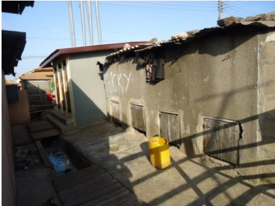
Figure 10-26 Toilet blocks in Nii: six VIP toilets (left) and four closed bucket toilets (right)
