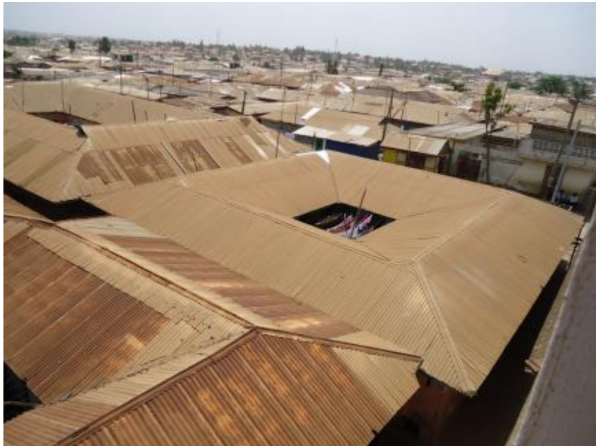
Figure 10-17 Houses and roofing in Nii
