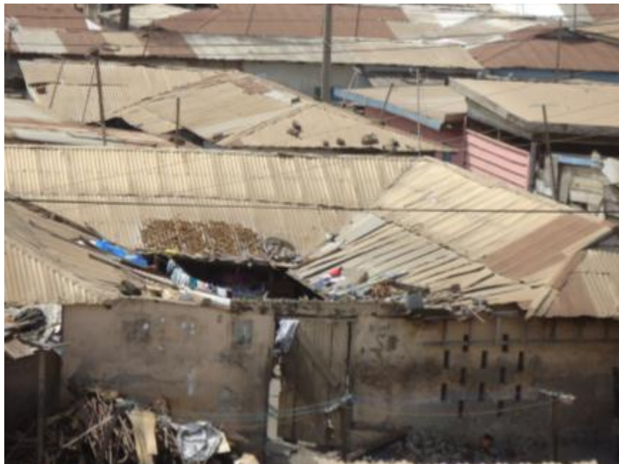
Figure 10-13 Compound houses in Nii
