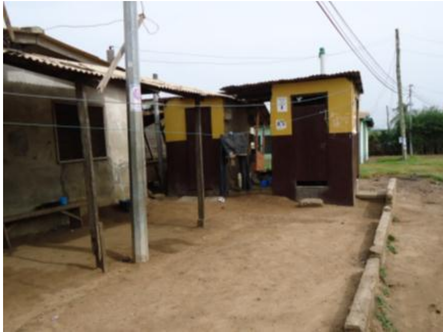
Figure 10-24 Neighbour shared toilets in Amui
