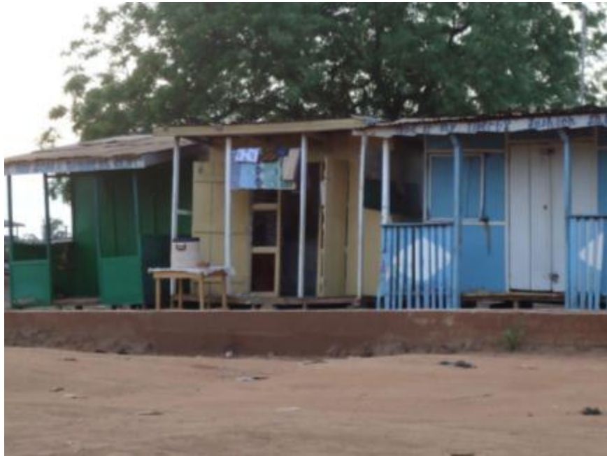
Figure 10-12 Wooden kiosks also used as bedroom at night-time
