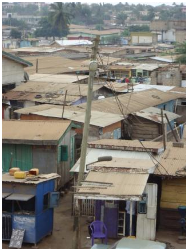
Figure 10-15 Houses and roofing in Amui
