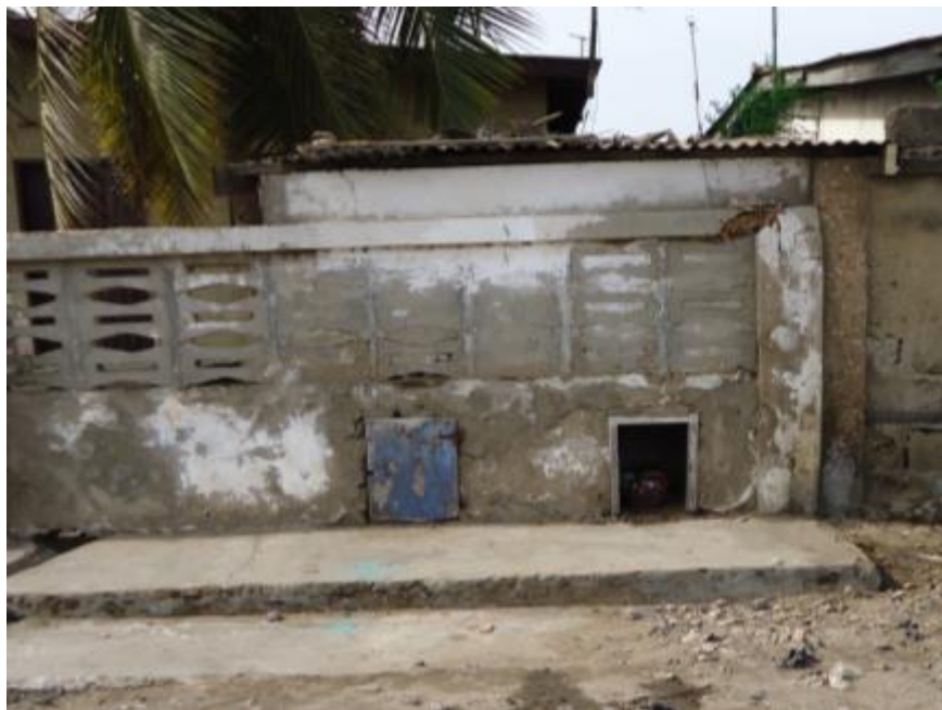
Figure 10-19 Closed down bucket toilets of a self-contained house in Amui
