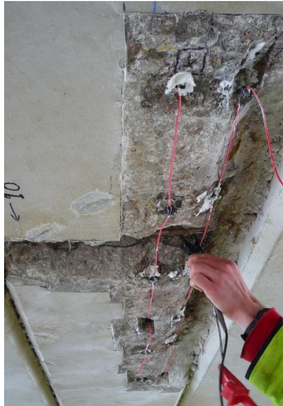
Figure 6: Hybrid anode installation on a prestressed concrete beam
