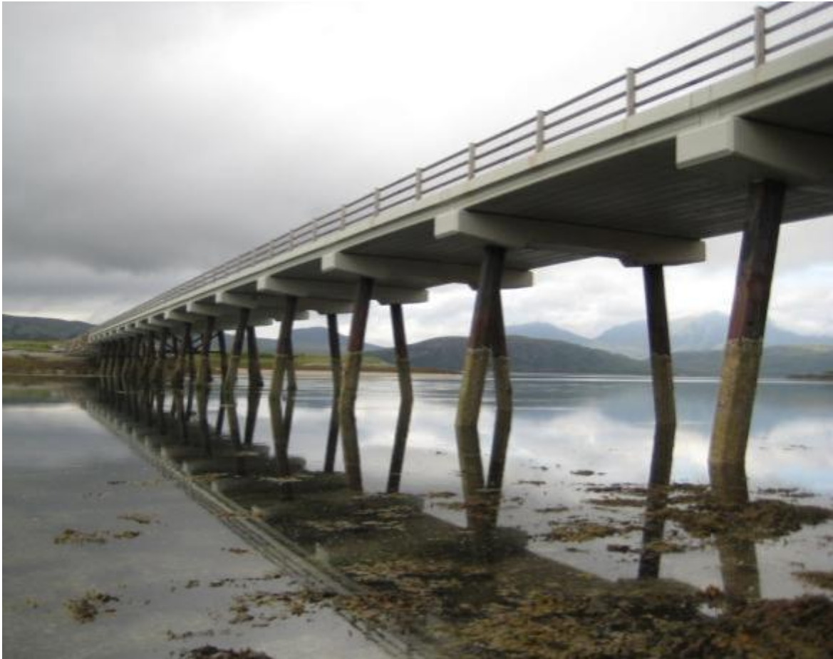
Figure 1: General view of the Kyle of Tongue bridge
