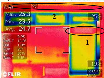
Figure 85. Internal infrared image of the house southern fenestration system
