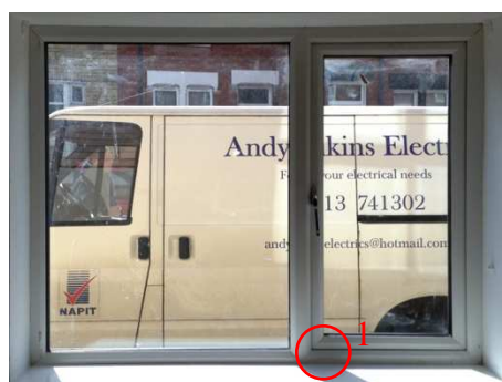
Figure 68. Internal photograph of west facing bottom flat window dwelling 7
