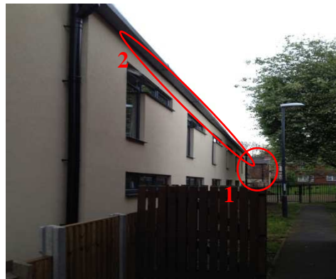
Figure 84. Photographic image of the southern elevation of the SHINE-ZC development.
