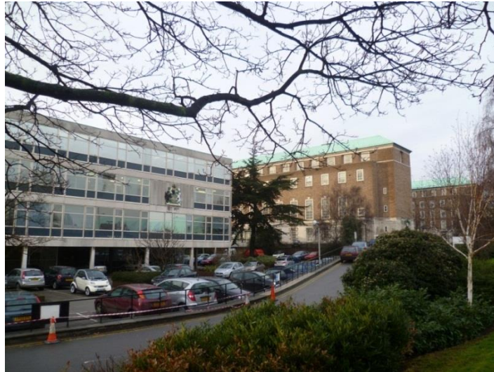
Figure 4.3 External view of the CLASP building (foreground) and County Hall (background)
