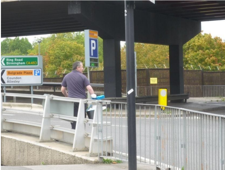
Fig 57; Potential consequences of deviation of safe pedestrian route from desire line
