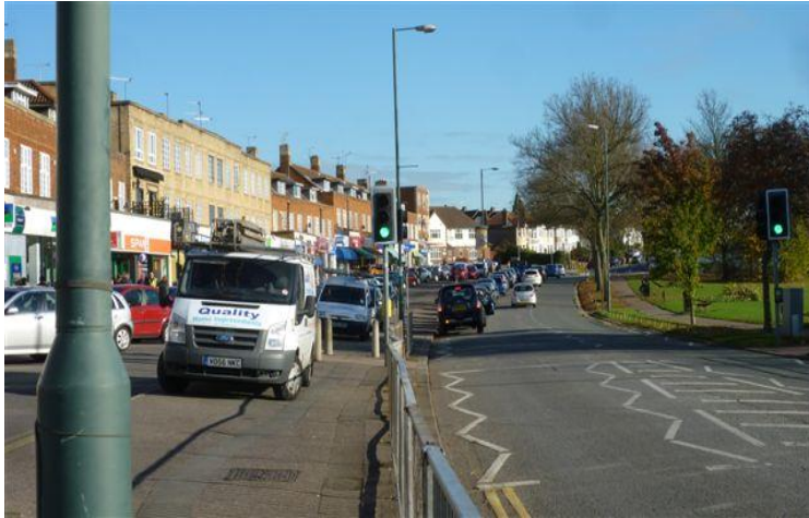
Fig 108; Pavement obstructions Daventry Road
