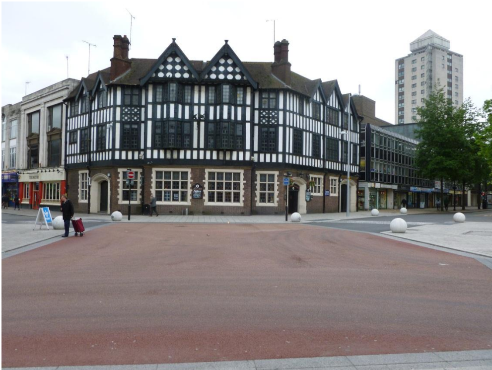
Fig 161; Junction of The Burgess, Hales Street and Bishop St, after creation of shared space scheme
