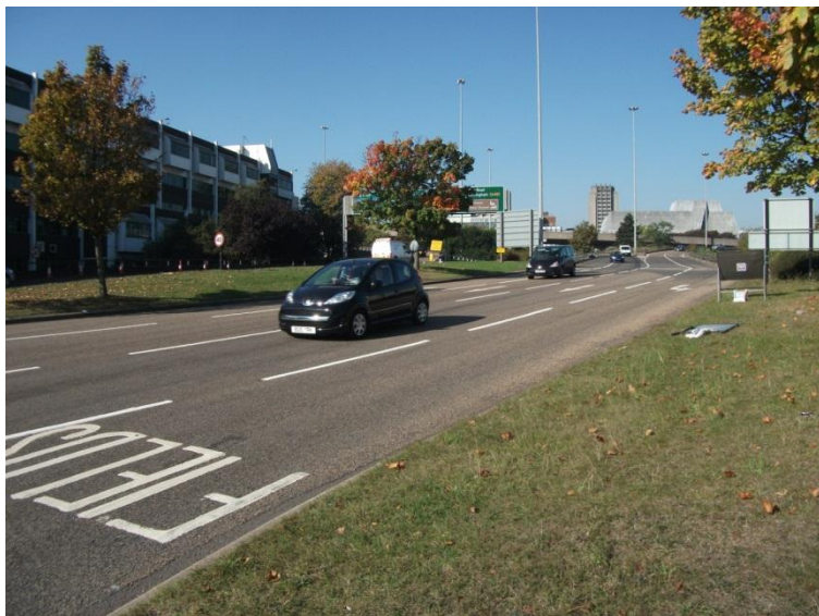
Fig 53; View of top exit slip road at Gosford St
