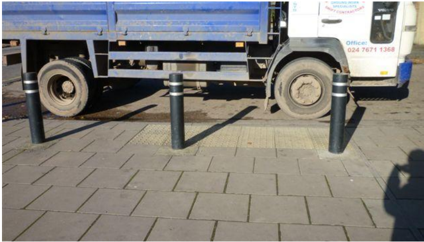
Figure 111; Parked vehicle obstructing the dropped kerb, Daventry Road
