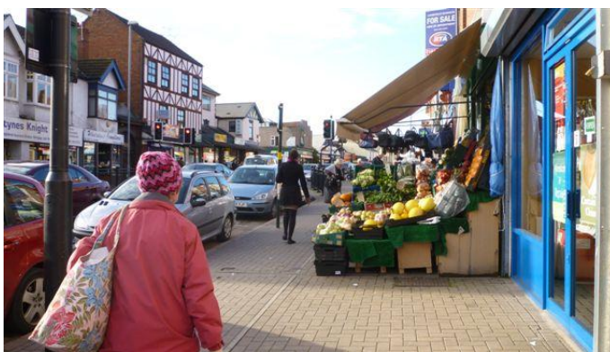
Fig 121; Pavement condition, Walsgrave Rd (1)
