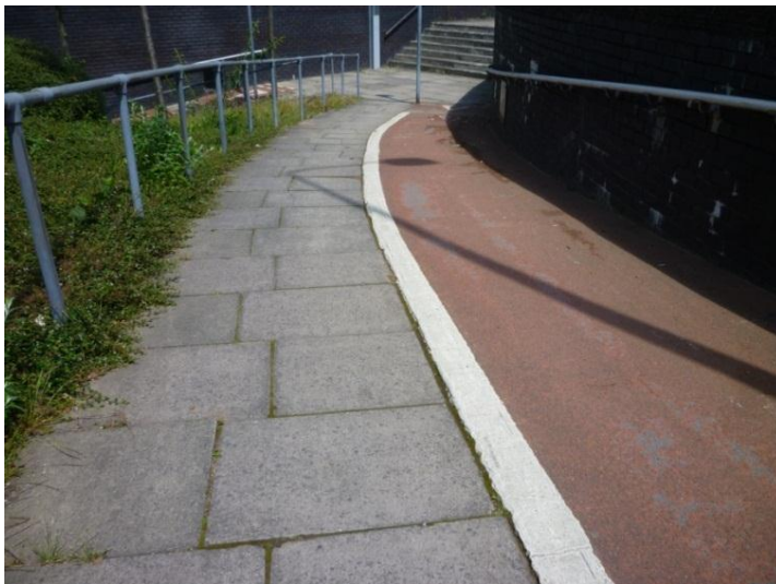
Fig 62; Subway access via a ramp, showing shared cycle/pedestrian pavement.
