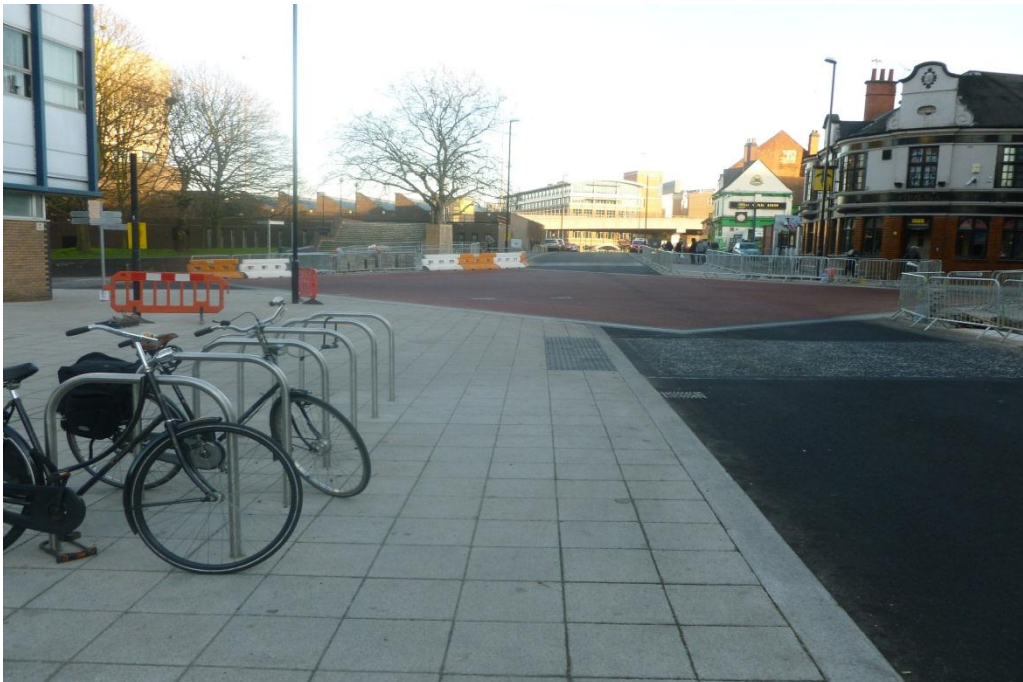
Fig 163, Junction of Fairfax St and Gosford St after shared space scheme
