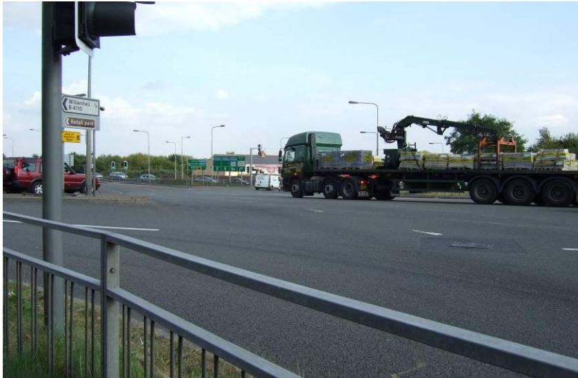
Fig 28; Toll Bar End roundabout
