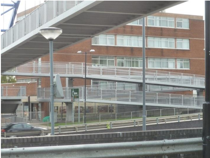
Fig 63; Over-bridge at Hill Street, showing length of the ramp access
