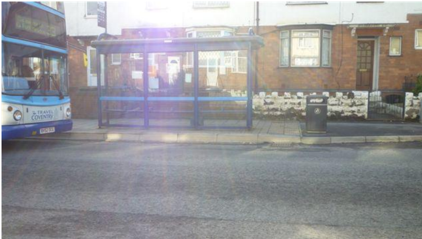
Fig 123, Raised bus kerb on Walsgrave Rd
