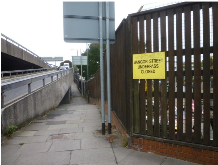
Fig 72; poorly signed pedestrian route
