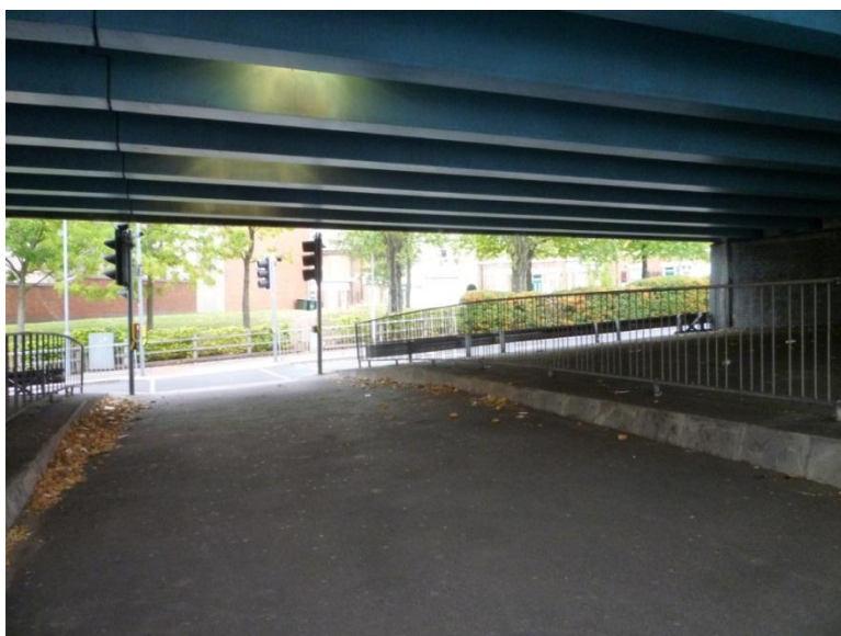
Fig 82; Poorly lit crossing point close to Albany Road
