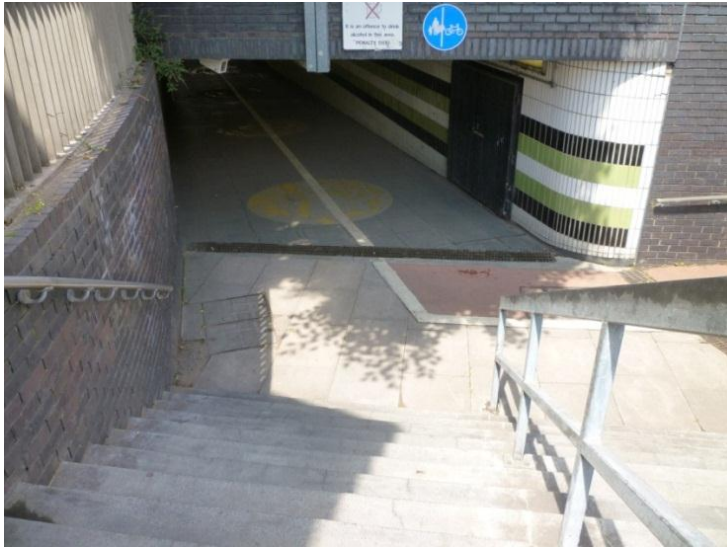
Fig 61; Subway access via steps
