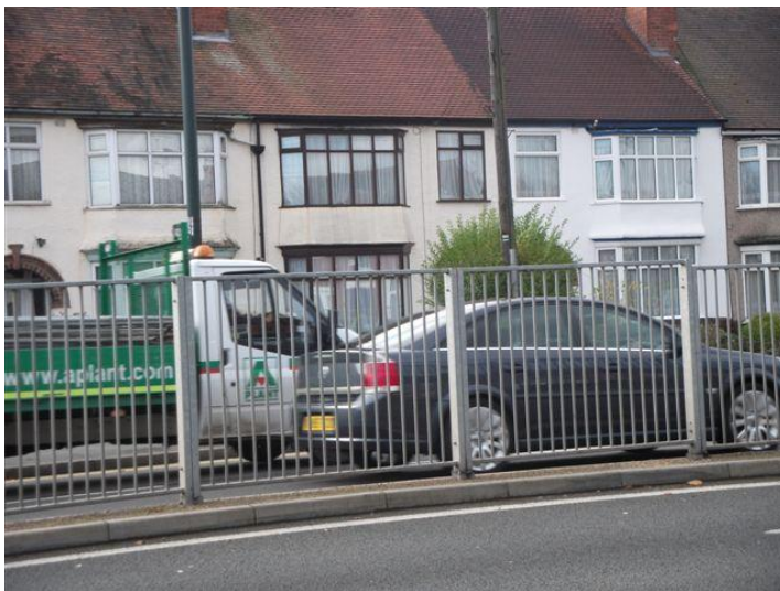
Fig 98; Kenpas Highway showing traffic and guard rail
