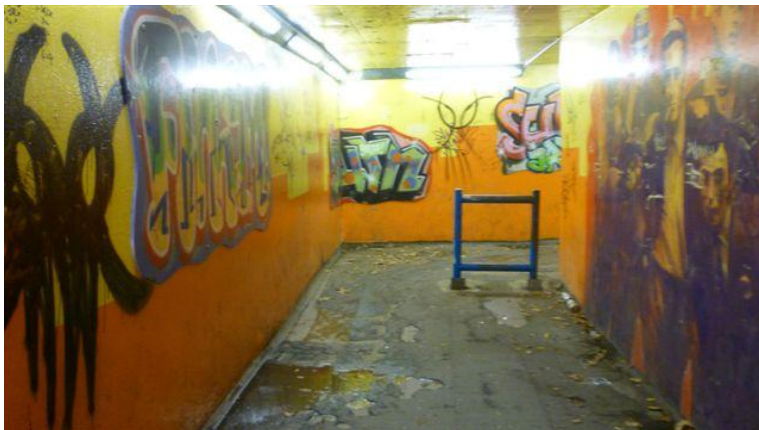
Fig 101 Kenpas Highway, subway
