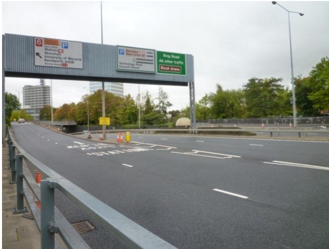
Fig 51; View of exit slip road at Railway Station – bottom of ramp
