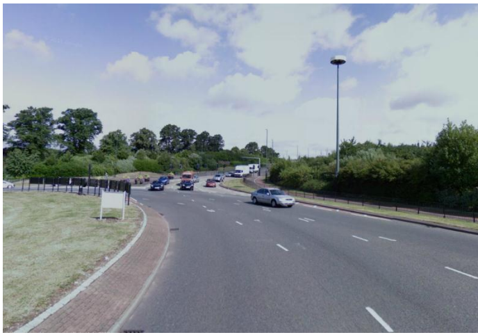
Fig 38; A444/Binley Rd, pictured from Binley Rd
