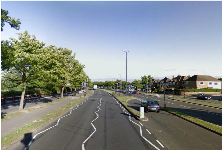
Fig 100; Kenpas Highway, at-grade crossing
