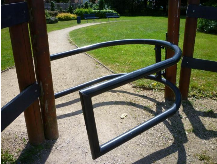
Fig 75; Obstruction to the footpath caused by street furniture
