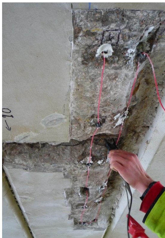
Figure 6 Typical hybrid anode installation on a prestressed concrete beam
