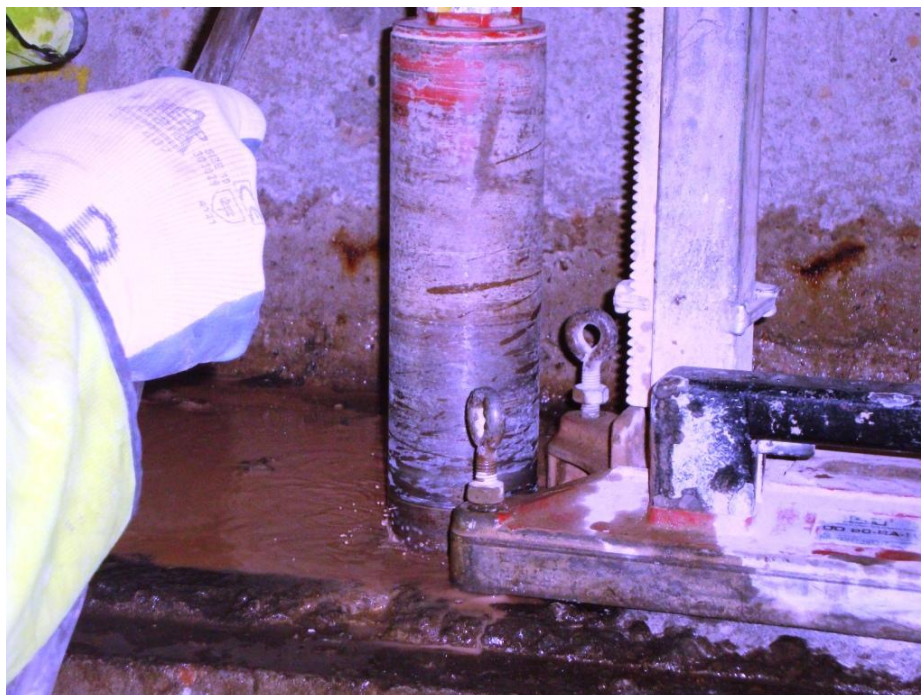
Figure 5: Coring on top of a silane-treated RC cross-beam
