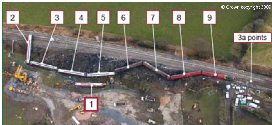
Figure 8 – Aerial view of the derailed train (numbers represent train vehicle number) (from RAIB (2011))
