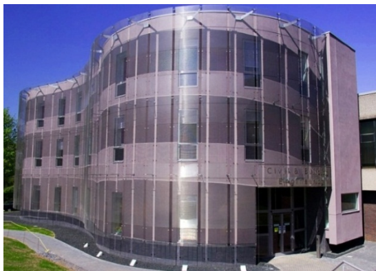
(a) Case study building
