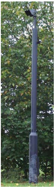
... and CCTV masts.
