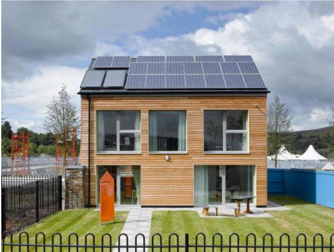
Figure 8 The 'Larch' Passivhaus Ebbw Vale (Jefferson Smith)
