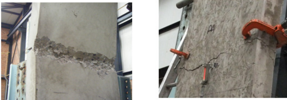
Figure 4.3 Panel Buckling Failure: (a) Unconfined Central Welded Mesh; (b) Welded Mesh with a 50\text{kg/m}^3 SFRC Content
