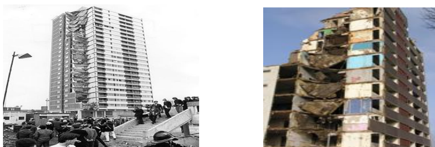
Figure 1.1 Disproportionate Collapse of Precast Cross-wall Structures: Ronan Point (1968) and Large UK Panel Structure during Demolition (CROSS 2000)
