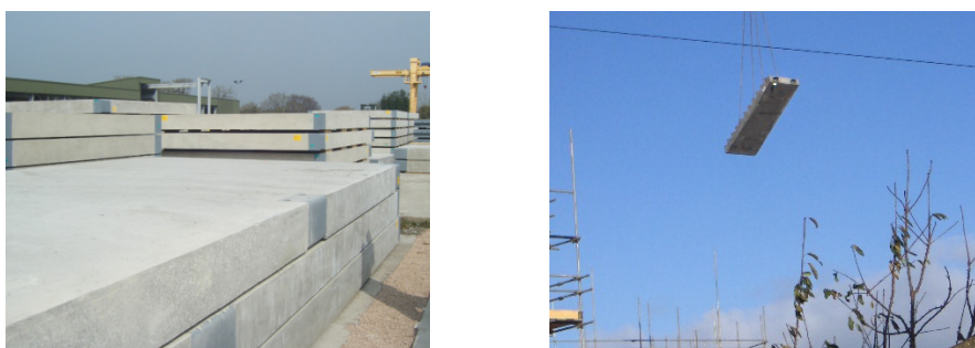
Figure 1.4 Large Scale Precast Flooring Units and Significance of Transport and Craneage Considerations in Precast Buildings.
