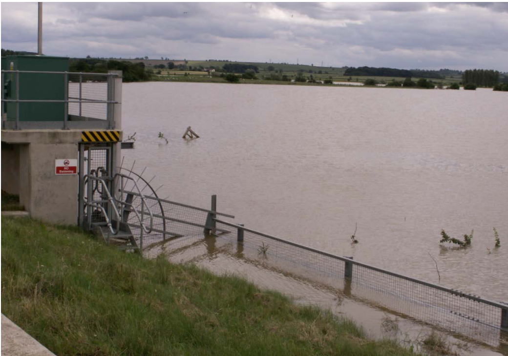
Plate 7.1 Photographs (courtesy of Julia Hawley), providing an indication of the extent and severity of the August 2007 flooding; i) shows the closed gates of the flood control structure taken from sampling location 3, ii) view from the earth dam of the flooded pastoral field.
