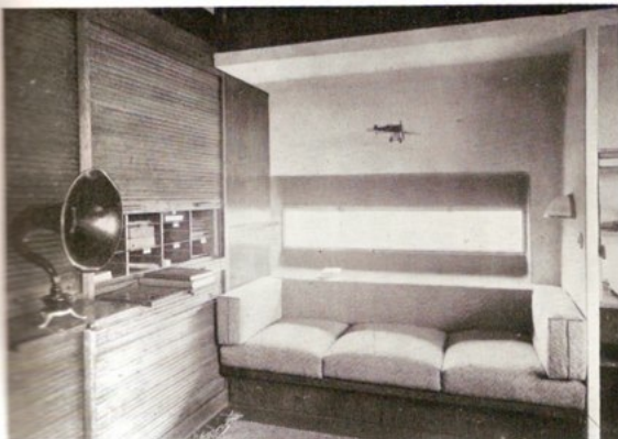
THE STUDY (24 on plan) has built-in furniture, bookshelves and filing cupboards, protected from dust by roll-shutters.
