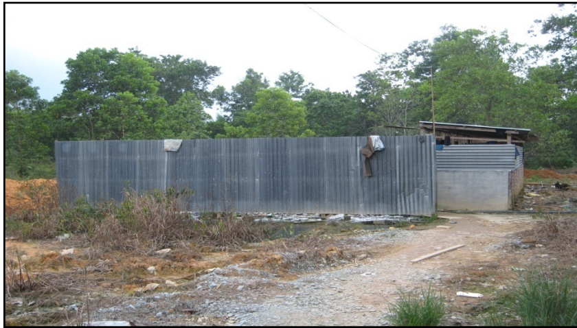
Temporary toilets and shower
