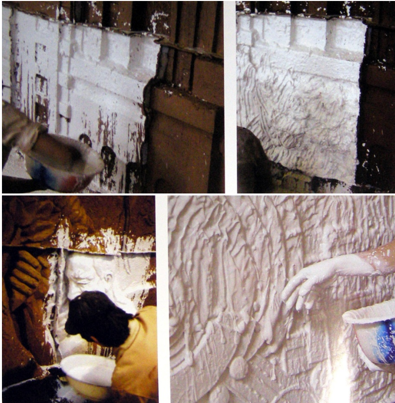
Figure 4-4 Applying plaster on the divisions of clay original
