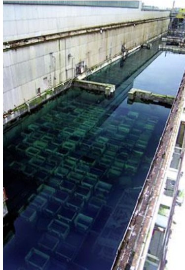
Figure 7. Photograph of a Magnox storage pond at Sellafield
