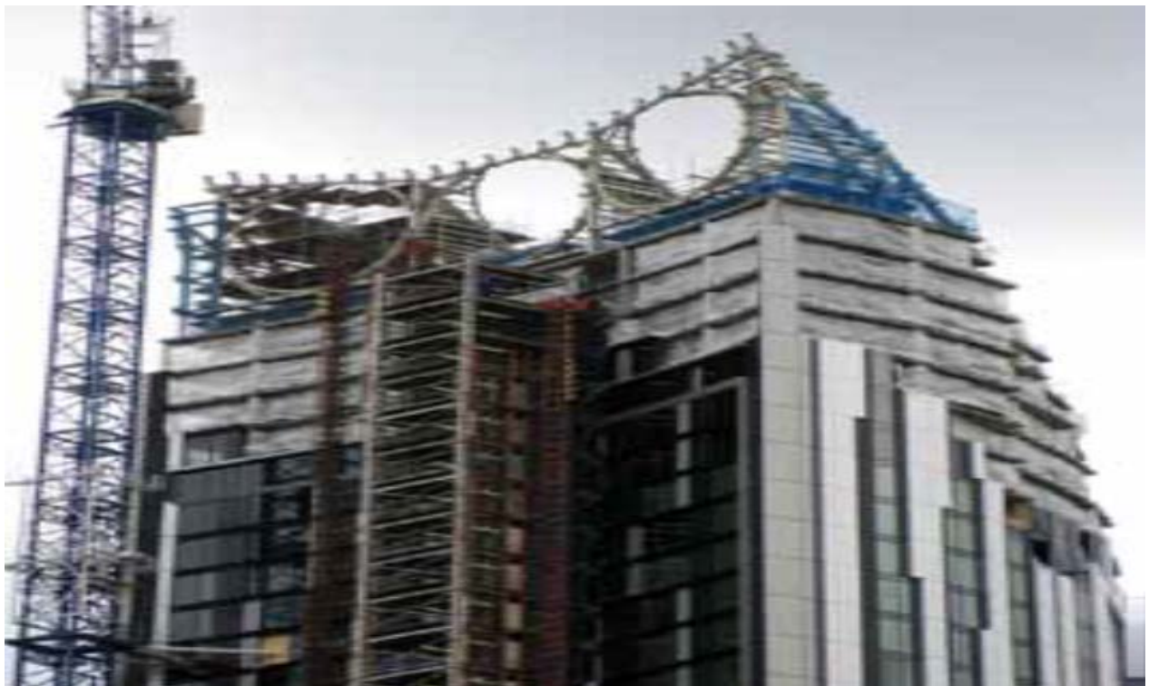
Figure 6.10 Site installation of the wind turbine enclosure panels
