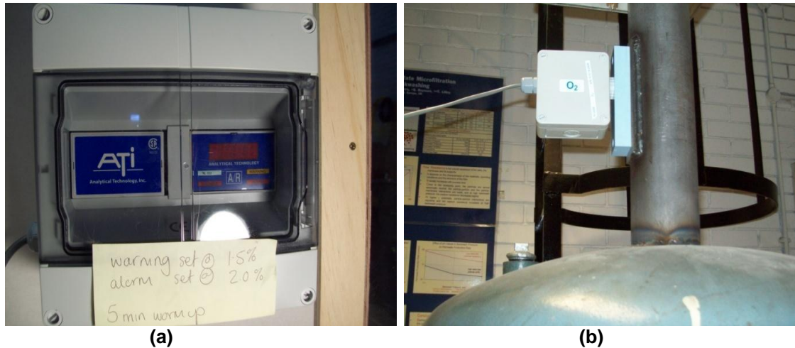
Figure 4-10: Gas/Oxygen Detecting System (a) Control Setting + Alarm Module and (b) Sensor/Transmitter Module
