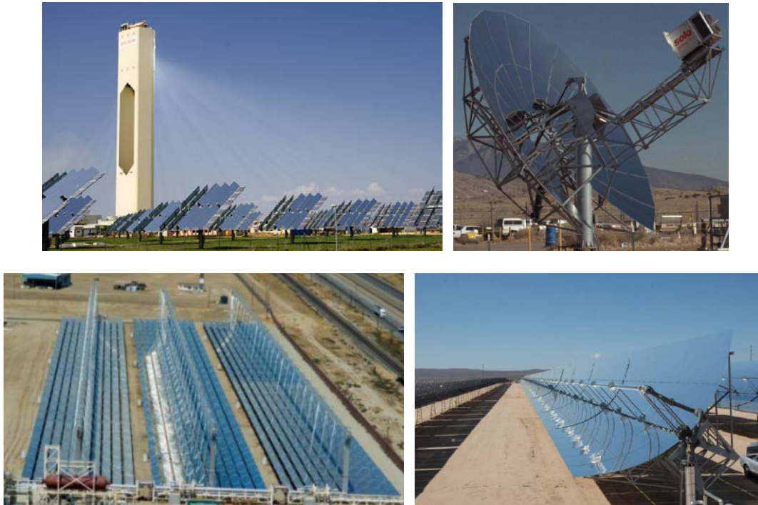
Figure 1: Four main commercial types of CSP plants: Abengoa Solar’s PS10 power tower, Seville, Spain (Top left) (Abengoa Solar, a, 2010); Flagsol parabolic troughs at Kramer Junction (SEGS V), California, USA (Bottom right) (Kearney, 2007); Sandia 10-kWe dish/String system (Top right) (Kearney, 2007); Linear Fresnel Reflectors at Kimberlina Solar power station, California, USA (Bottom left) (Areva Solar, 2010).
