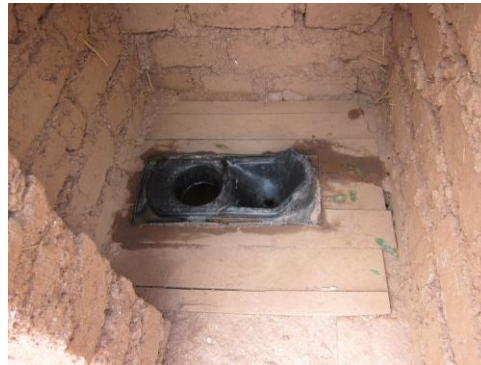
Two views of the replacement semi-ecosan latrine built with support from an NGO (Photo: Author, Rwanda, 2012)
