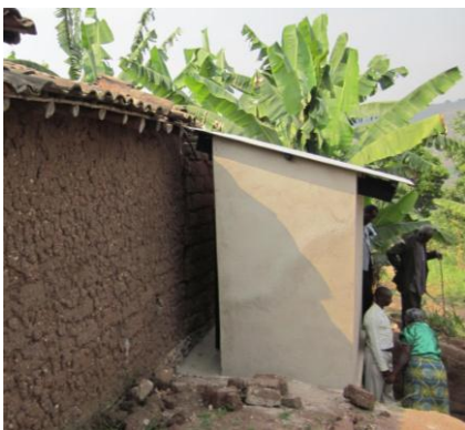
Two views of a double vault ecosan latrine built by and NGO in the western province (Photo: Author, Rwanda, 2012)
