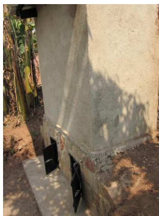
Two views of a double vault ecosan latrine built by and NGO in the western province (Photo: Author, Rwanda, 2012)
