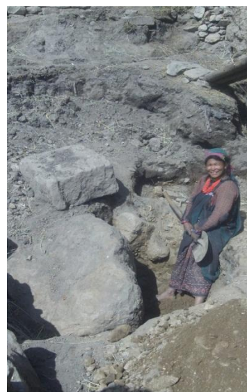
Figure 8-5 A woman digs a latrine pit in very rocky ground
