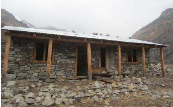
Figure 6-22 A healthpost building in Chaggaunphaya that was never staffed (Author, 2012)
