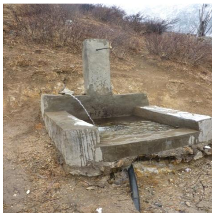
Figure 6-4 A typical cemented standpost. In this case with water arriving via a plastic pipe held by a stone to the left of the main body of the tap with the main outlet redundant (Author, 2012)
