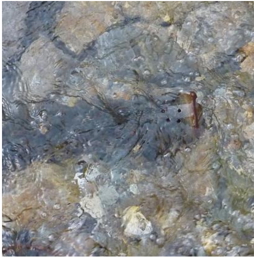
Figure 6-2 An intake from a river using unprotected perforated piping (Author, 2012)
