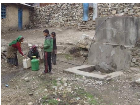
Figure 6-25 Tap at Chaggaunphaya school with attached reservoir (Author, 2012)
