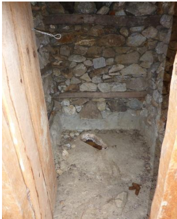
Figure 6-18 A filled latrine pit (one of two) by Kermi hot springs (Author, 2012)
