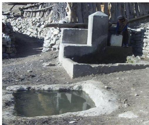
Figure 6-26 Drainage from a tap feeds into a small pond for animals in Chaggaunphaya
