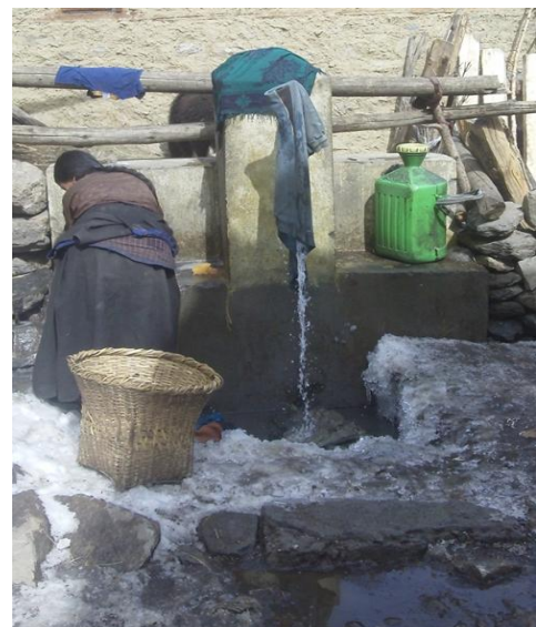
Figure 7-3 A woman uses a tap with poor drainage resulting in water freezing in its apron (Author, 2012)
