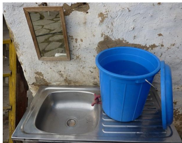
Figure 6-11 Handwashing facilities in the Nepal Trust Guest House in Simkot (Author, 2012)
