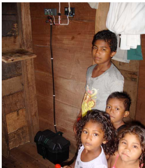
Figure 25. Batteries are transported to users and connected to home kits
