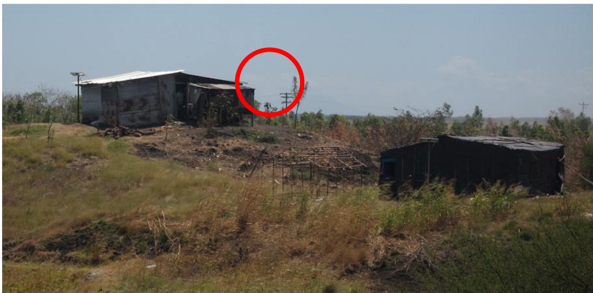
Figure 28. Overhead power cables in Chiquistepe - but no connections
