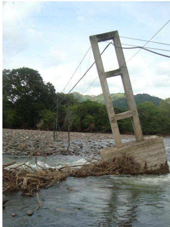
Figure 8. Foot bridge destroyed by heavy rains during 2011, preventing access to the community of San Ramón (Condega, Estelí)
