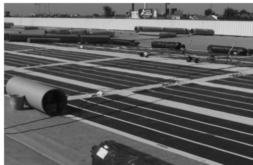
Figure 1: Triple junction amorphous modules during installation in Seville.
