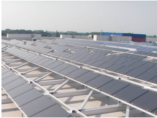
Figure 1: Photograph showing micromorph PV modules on the Gent store.
