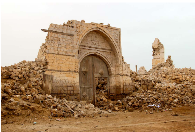
Figure 2. Deterioration of Suakin's historic coral block buildings
