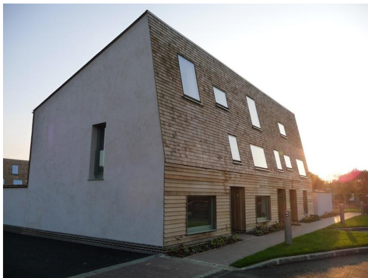
Figure 4- 1 Elmswell - Energy efficient residential development (Buro Happold, 2009)
