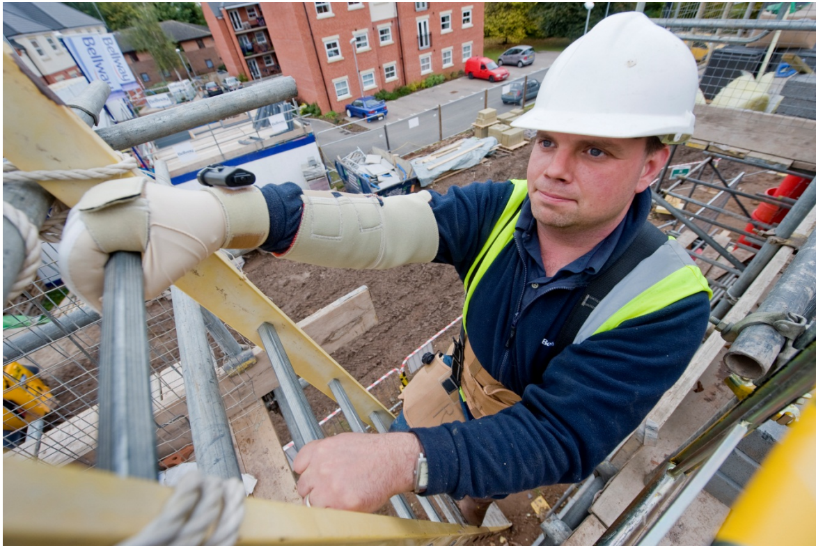
Figure 3 Worker climbing ladder wearing upper limb disorders and HAVS simulations
