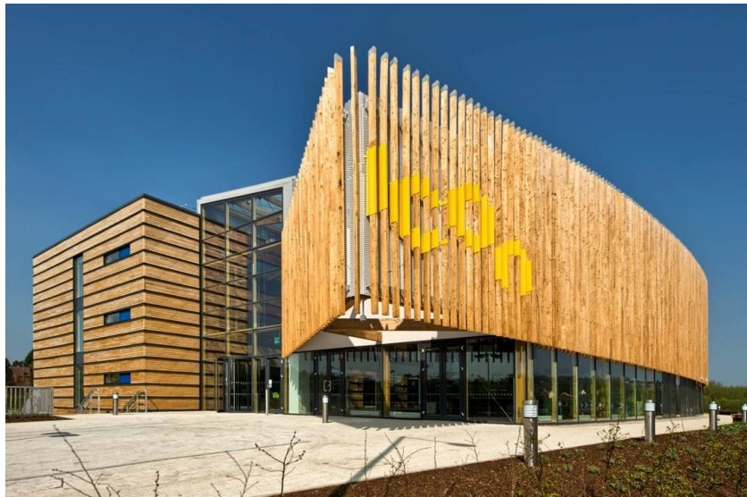
FIGURE 3.1: South façade showing café, street and incubator office block
