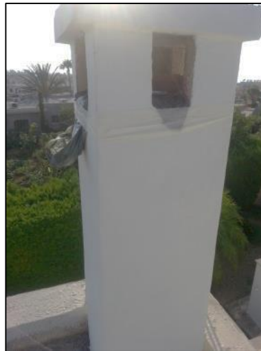
Figure C. 1 Sealing fireplace's chimney
