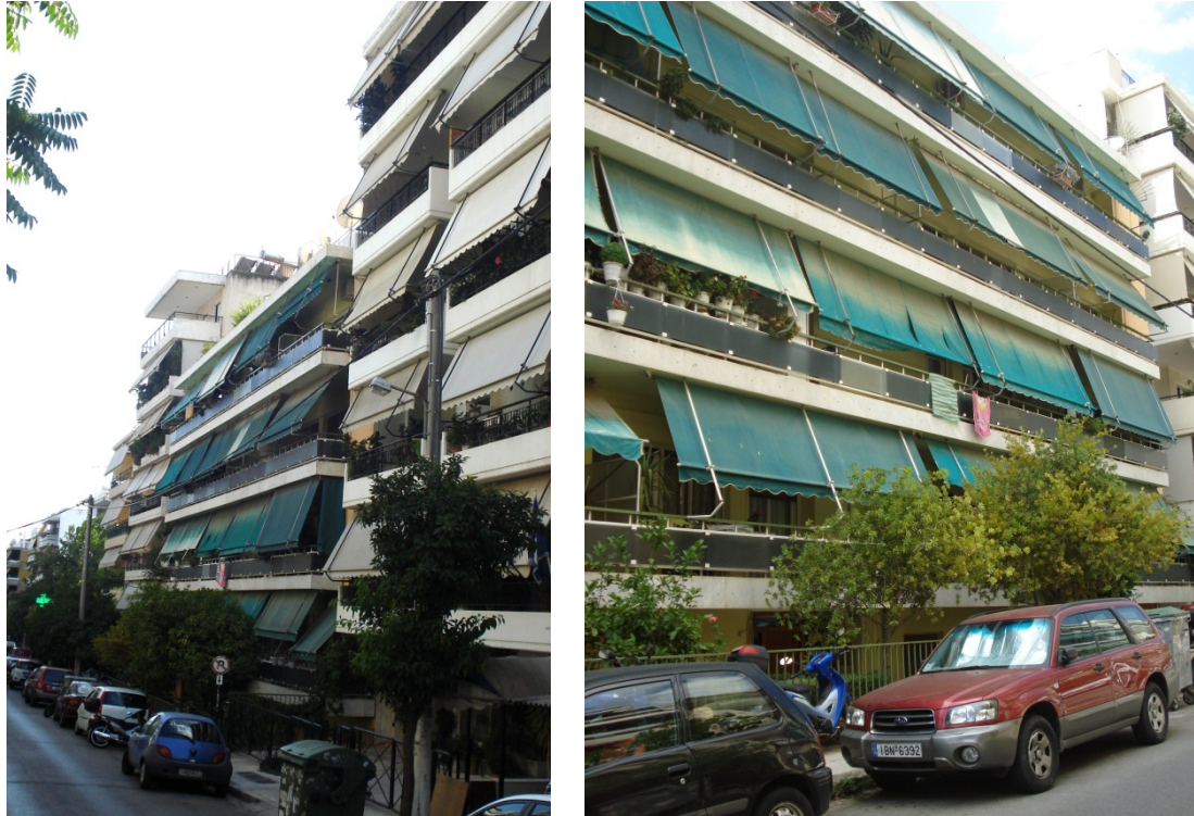
Figure 4.6 Views of the case study building (Photographs by author, 2012)
