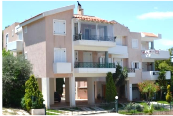
Figure 2.18 Modern apartment building with pilotis used for parking area in Saronida, Greece (photograph by author, 2012)
