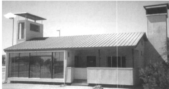
Figure 2.26 Test building with an evaporative cooling chimney (left) and a tower (Givoni, 1998)
