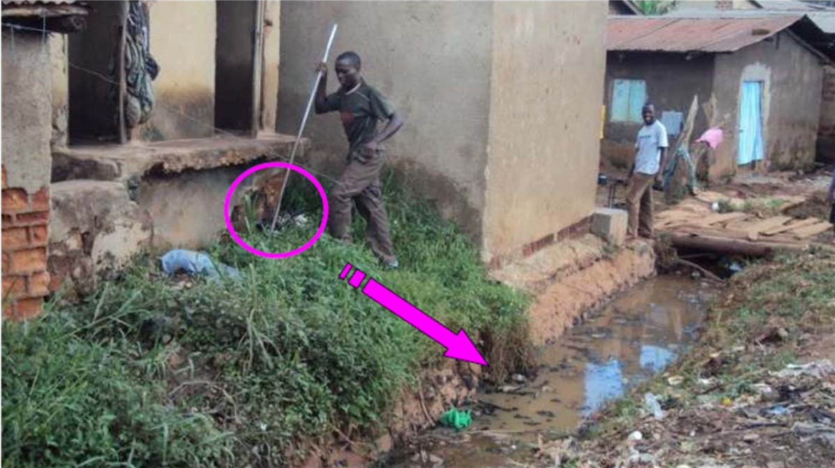
Fig.1.4 Sewer pipe vandalization and release of slurry into immediate environment [adapted from (20)]
