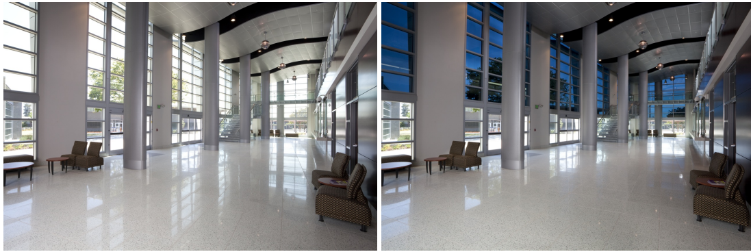
Figure 1 – Images showing electrochromic glazing in clear and darkened state (photos courtesy SAGE Electrochromics Inc.)
