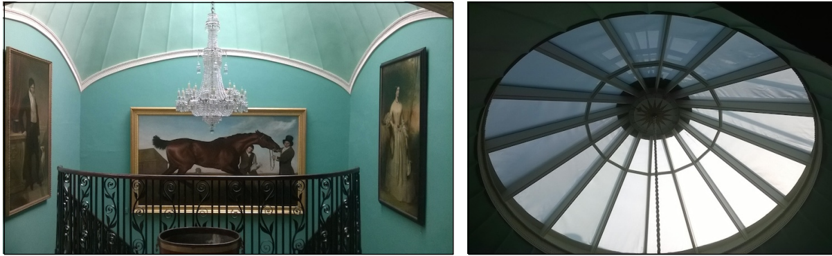
Figure 6 – Photographs of the Stone Staircase and rooflight following the interventions
