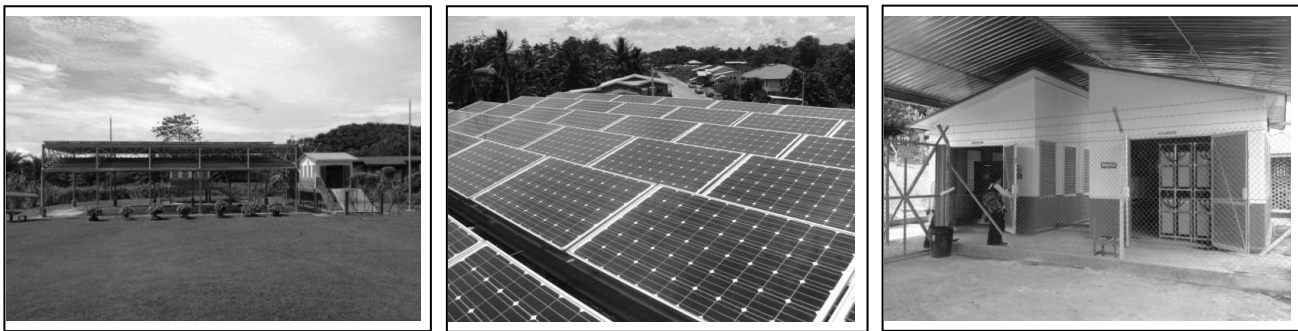
Fig. 3. (left) Solar PV structure and power house at SK Labuk Subur, (centre) solar PV panels at SK Sungai sungai, (right) system power house for batteries, inverters, diesel generator and other accessories at SK Lung Manis.
