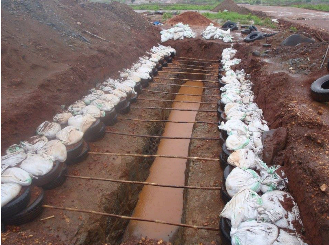
Figure 8 Recycling car tyres and using sandbags
