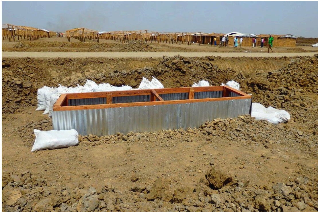
Figure 6 Trench latrine under construction
