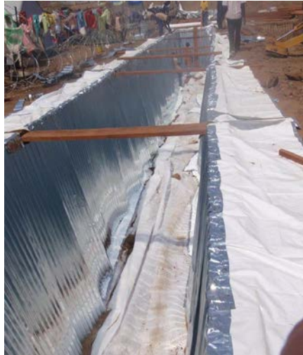
Figure 2 Trench latrine under construction; this collapsed later
