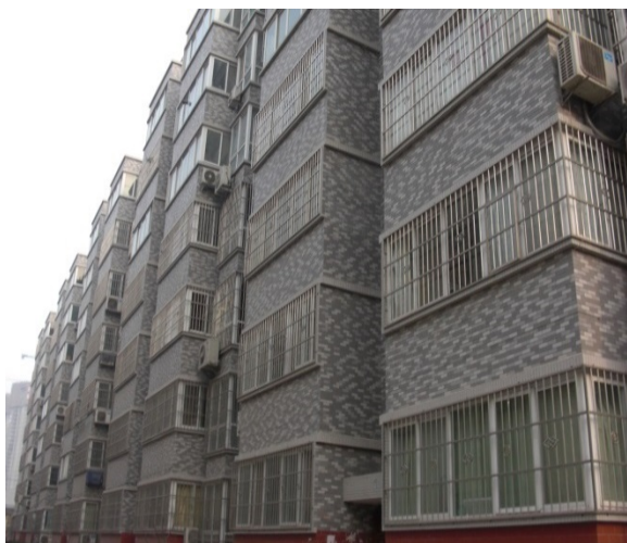
Figure 2 (b) photo of monitored new building
