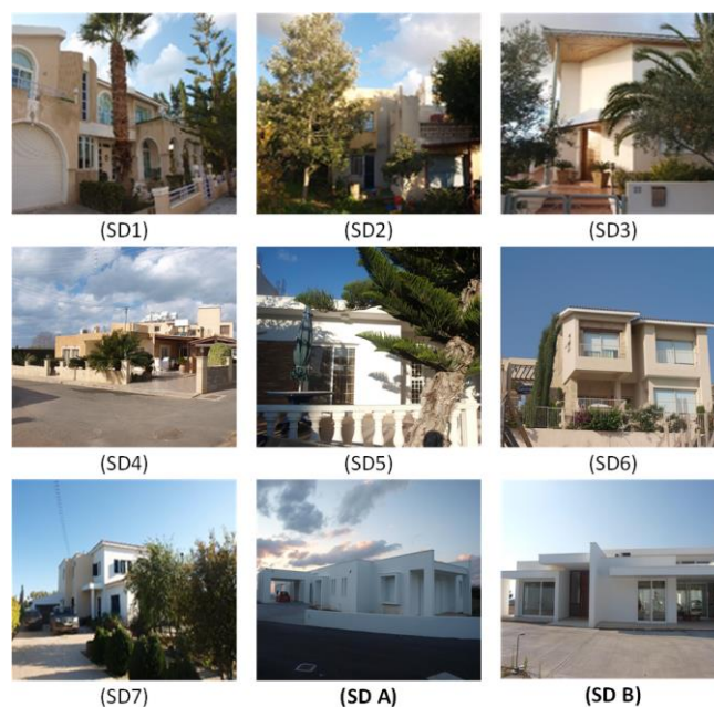
Figure 2 Exterior view of case studies
