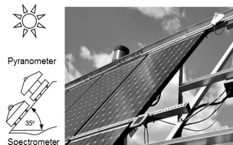
Fig. 7 Outdoor PV performance and meteorological data monitoring system.
