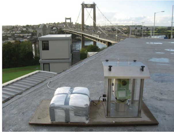
Figure 2.3: Robotic total station at Tamar Bridge (Battista et al. , 2011).
