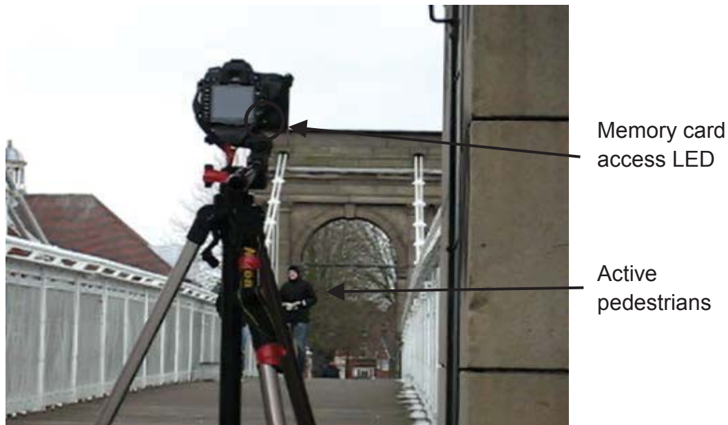
Figure 4.12: Freeze frame from the video camera of the Wilford Suspension Bridge during test
