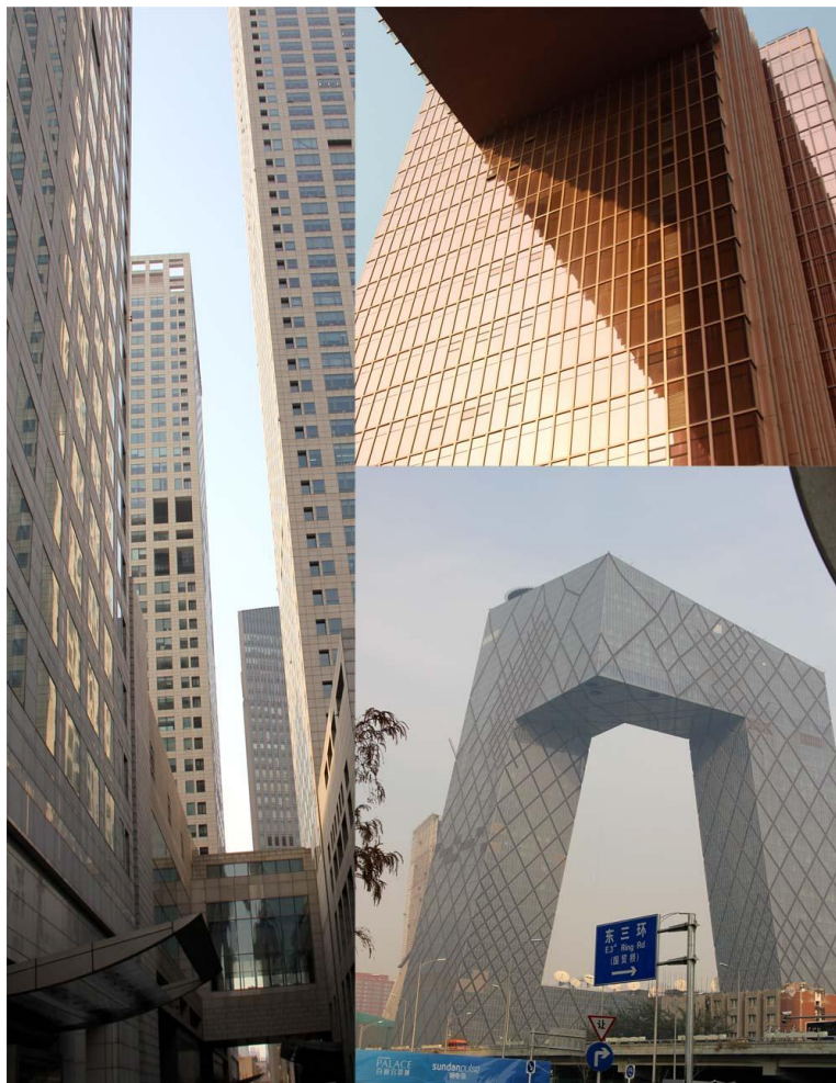
Figure 4.7 The skyscrapers of the CBD in Beijing.
