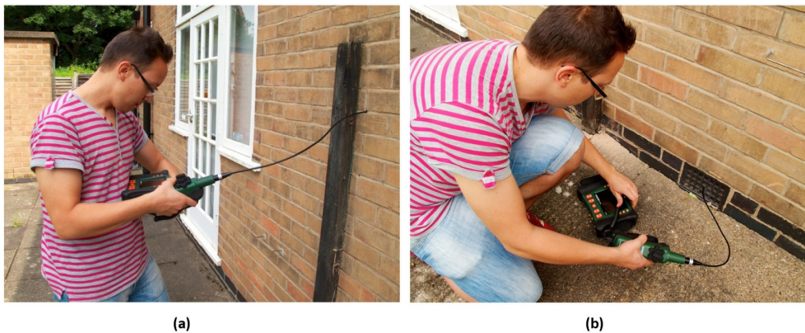
Figure 3-8: Borescope investigation at the test houses: (a) exploring external wall cavity; (b) exploring subfloor construction through air bricks ( Photos by Stephen Porritt )
