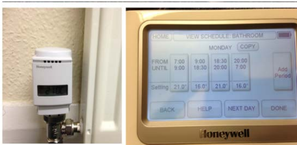
Figure 4-6: A PTRV installed on a radiator (on the left) and the interface of the central controller used to programme the PTRVs (on the right)
