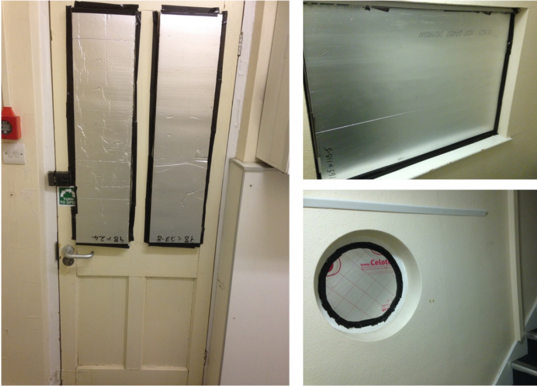
Figure 3-3: The West facing windows in the House 1 which were covered by 50 mm PIR insulation boards
