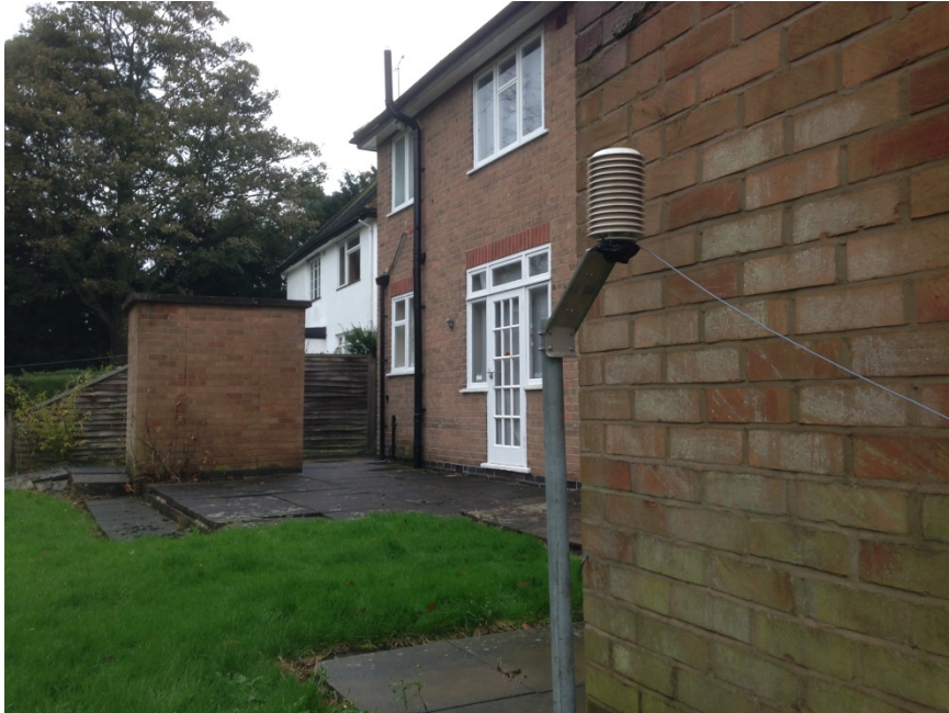
Figure 4-3: The location of temperature sensor used to measure outdoor air temperature and its shielding
