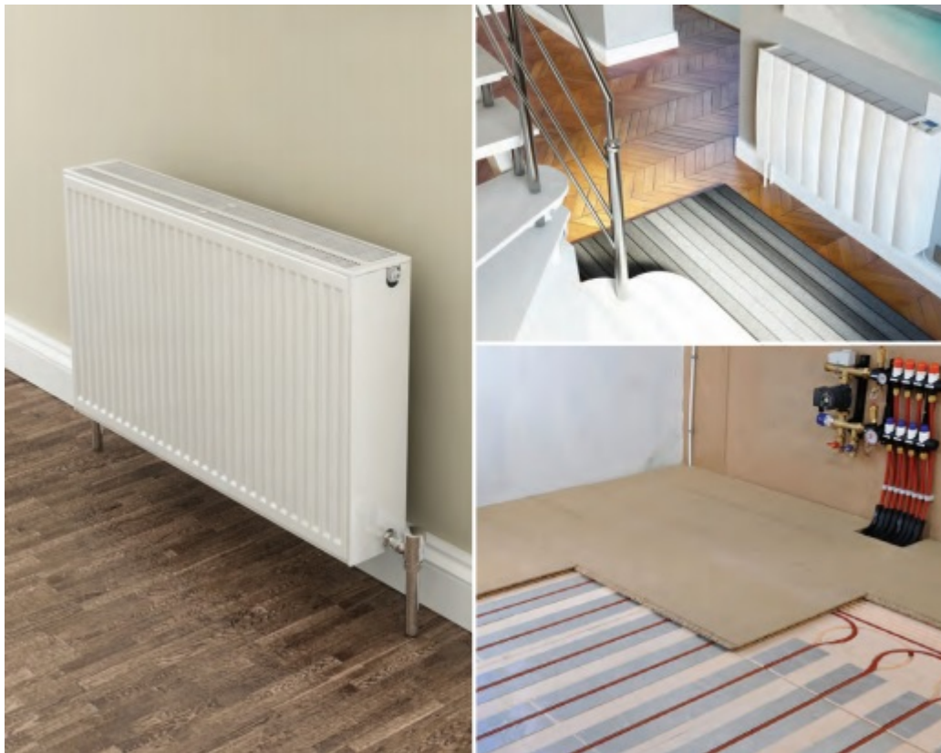
Figure 2-8: Three common types of heat emitters: panel radiator, fan convector and underfloor heating coils (Young et al. 2013)
