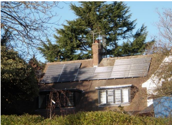
Figure 5: Shading by a Nearby Tree Example (Credit: Brian Goss, CREST)
